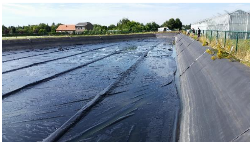
Figure 4-14 Installing a floating cover for a rain water storage.
